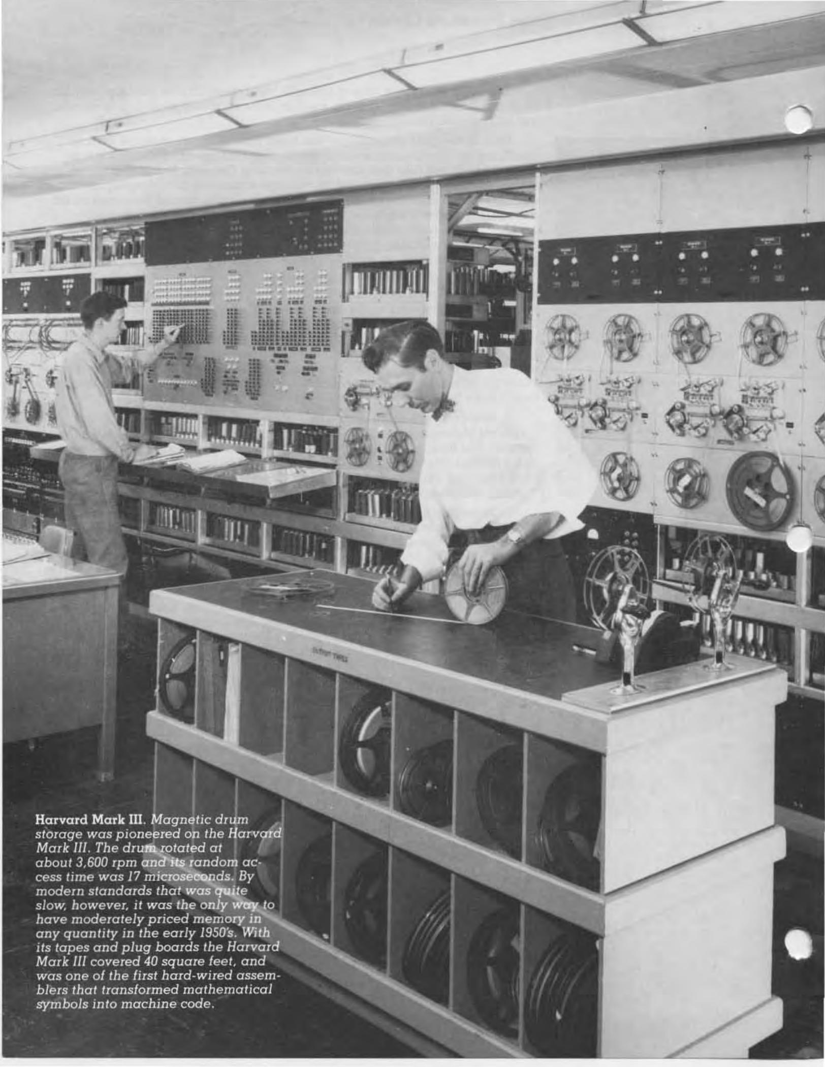
**Harvard Mark III.** Magnetic drum storage was pioneered on the Harvard Mark III. The drum rotated at about 3,600 rpm and its random access time was 17 microseconds. By modern standards that was quite slow, however, it was the only way to have moderately priced memory in any quantity in the early 1950's. With its tapes and plug boards the Harvard Mark III covered 40 square feet, and was one of the first hard-wired assemblers that transformed mathematical symbols into machine code.
