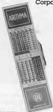
The Addiator was a very inexpensive and widely-sold pocket calculator. Introduced in 1920, over 100,000 were sold the first year. The Addiator was not truly mechanical in operation. The user added by sliding either up or down strips of metal with numbers marked on them. No gears or inter-linked parts were involved. The basic idea was first invented in 1889 by a Frenchman named Troncet. Troncet called his calculator the Arithmographe. From the collection of Gwen and Gordon Bell.
