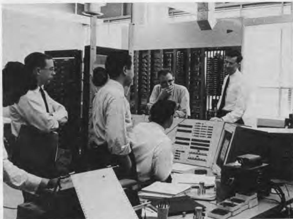
**Professor Jack Dennis:** Because the TX-0 was created as a memory test computer, it had some peculiar characteristics. The size of the address for the TX-2 memory was 16 bits, while the TX-0 had an 18-bit word. How do you build a machine with a 16-bit address and an 18-bit word size? Since an ordinary single-address instruction format was used, only two bits were left for the operation code.
