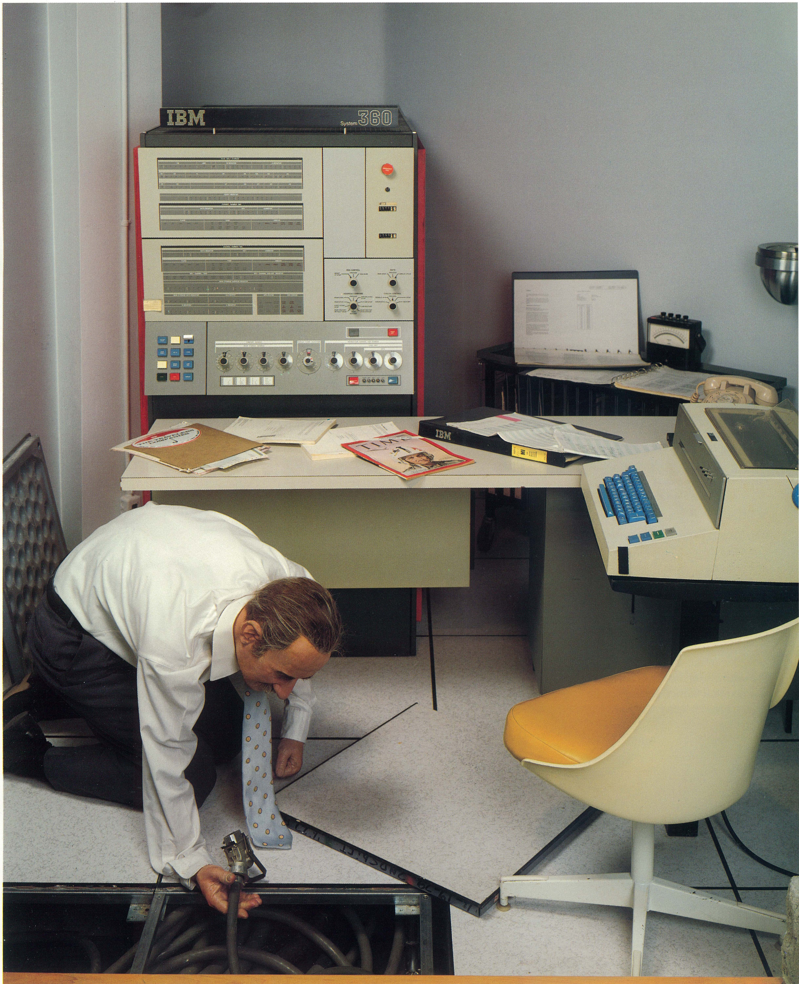
Mainframe computers required their own special facilities. Here, a technician installs cabling for a new tape drive.
