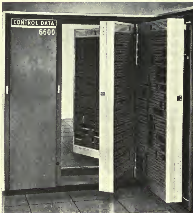
Fig. 9. 6600 main frame section.
